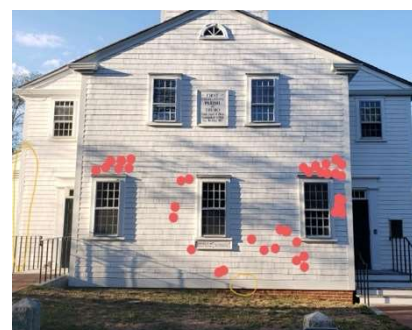
Evaluation of the rotted shingle siding by Tim Seaton, maintenance person/painter, 2020
