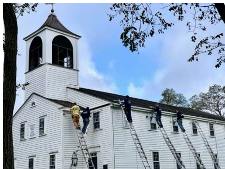
Replacing the gutters and repairing and painting the fascia boards, 2019.
