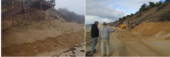
**Recommendation:** 1 cubic yd of sand per foot of shoreline, against the toe of bank This should be spread up the bank, planted with Beach grass and using biomimicry.
