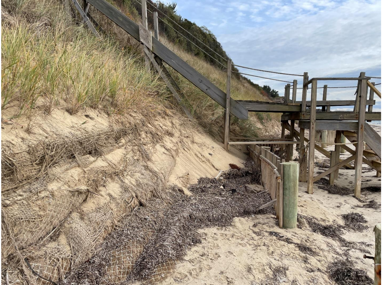
Figure 12: Image of the staircase at 17 Avocet Road. Degradation of the jute netting over the existing fiber rolls can be seen.
