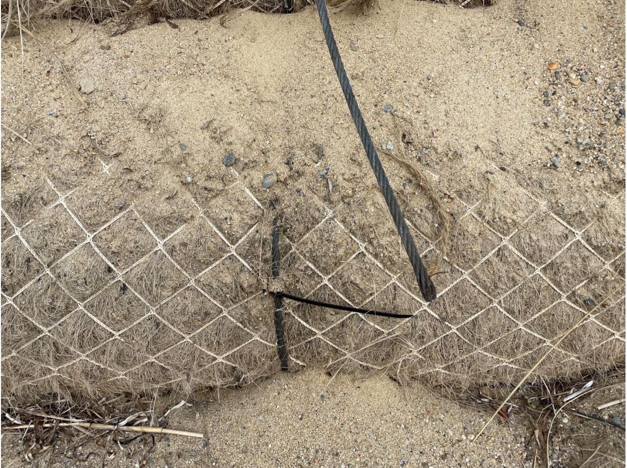
Figure 11: Image of the broken anchor cable for existing fiber rolls.
