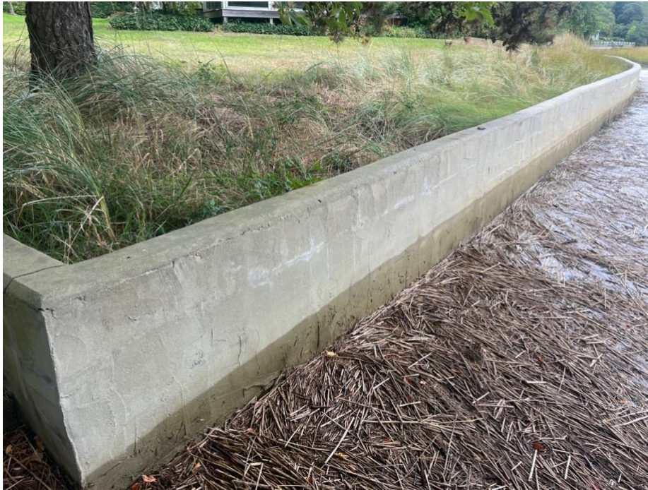
A SINGLE COURSE WOULD BE ADDED ON TOP OF EXISTING WALL
