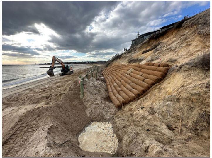
THE BOTTOM ROLL IS INSTALLED UNDER EXISTING GRADE TO PROVIDE A STRONG BASE AND PREVENT SLUMPING
