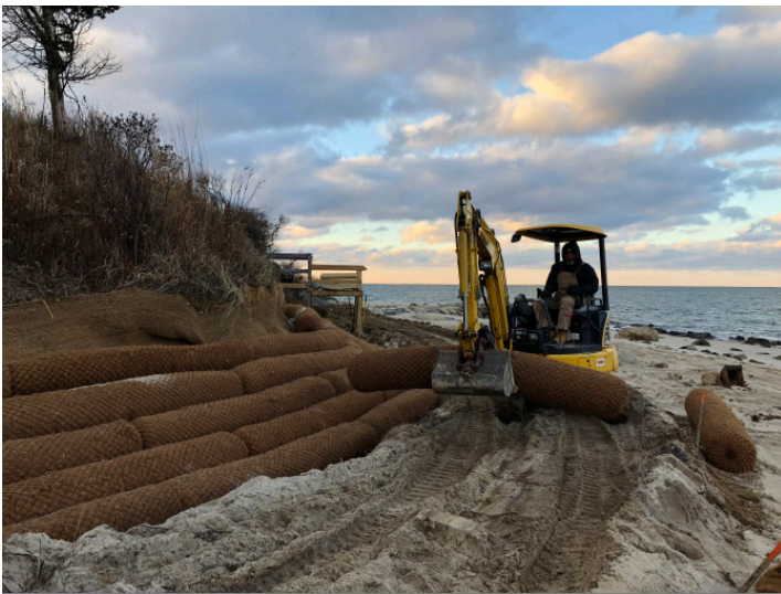
ROLLS ARE STACKED VERTICALLY ALONG THE FACE OF THE BANK TO RESTORE A DESIRABLE SLOPE
