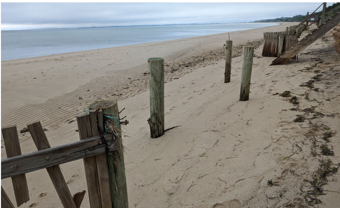
CONDITION OF EXISTING DRIFT FENCING; MANY PANELS ARE DAMAGED OR HAVE DISAPPEARED FROM THE SITE.
