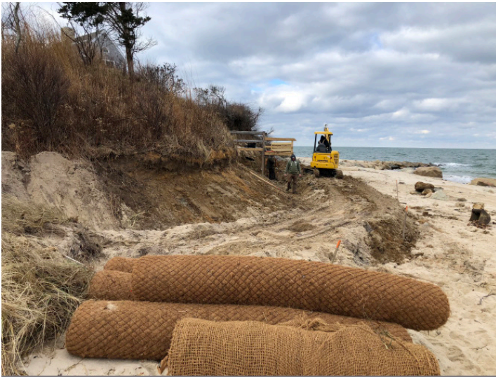
SLOPE IS PREPARED
