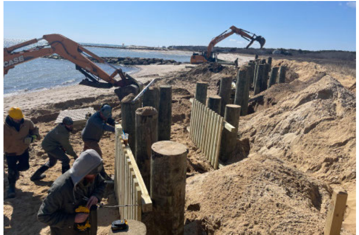
PANELS ARE ARRANGED IN A ZIG-ZAG FORMATION TO HELP CAPTURE WIND-BLOWN SEDIMENT
