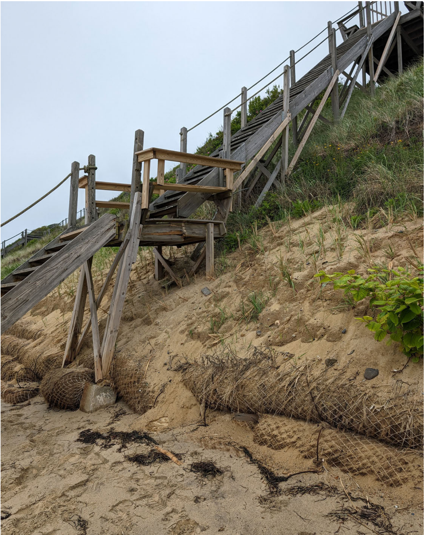
CONDITION OF EXISTING STAIRCASE, WHICH HAS BEEN DAMAGED AND IS NO LONGER SAFE TO TRAVERSE.
