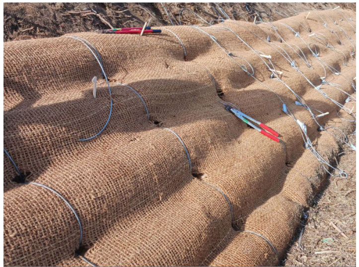
ARRAY IS BLANKETED AND ANCHORED IN PLACE
