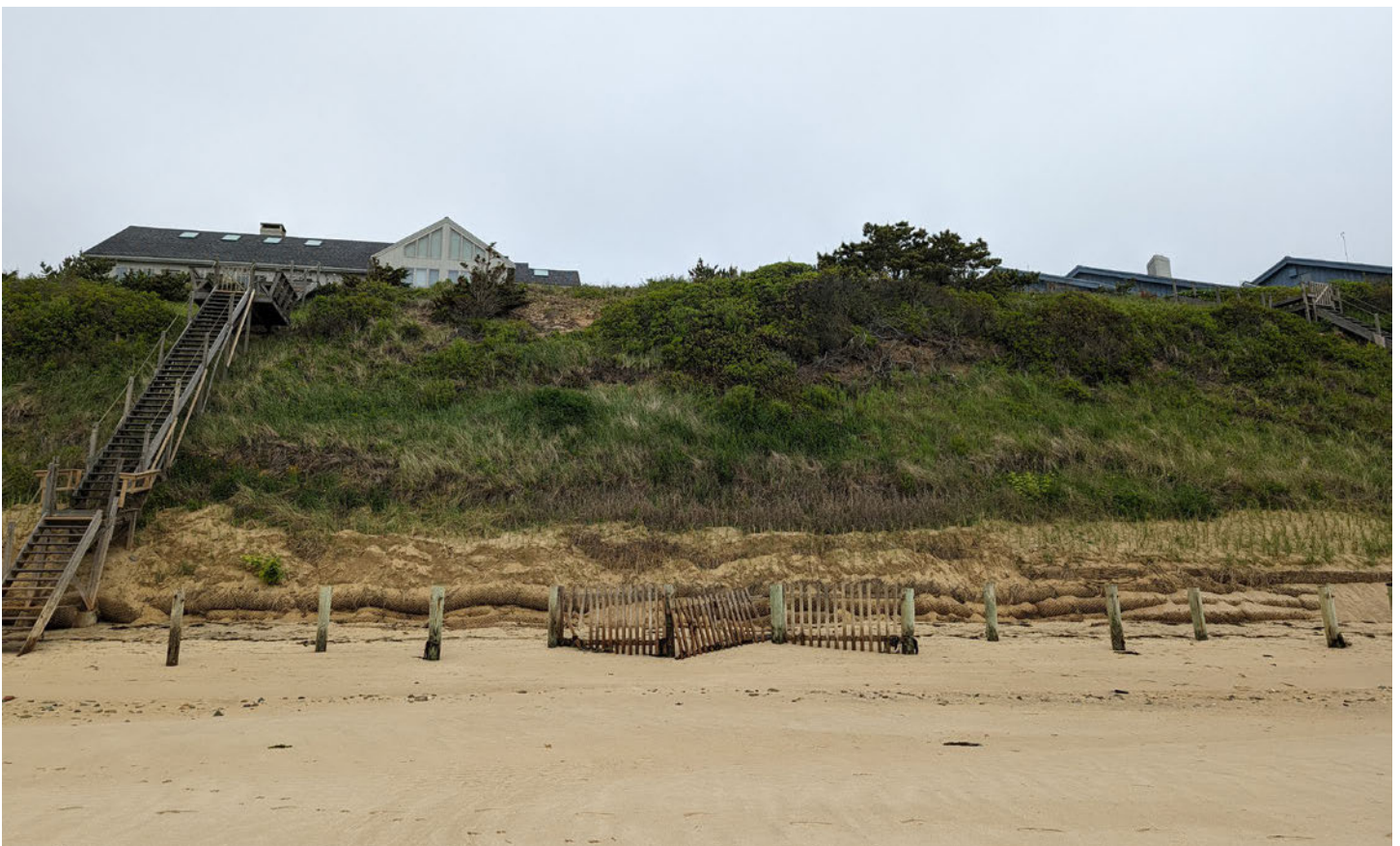
CONDITION OF EXISTING FIBER ROLL ARRAY, DRIFT FENCING, AND STAIRCASE AS SEEN FROM THE COASTAL BEACH.
