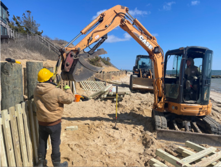
PANELS ARE ASSEMBLED AND LAID OUT
