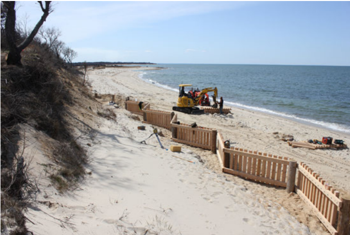
PANELS ARE ARRANGED IN A ZIG-ZAG FORMATION TO HELP CAPTURE WIND-BLOWN SEDIMENT
