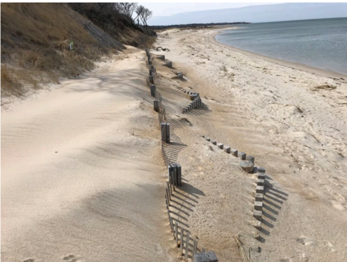
OVER TIME, THE FENCE ACCUMULATES WIND-BLOWN SEDIMENT
