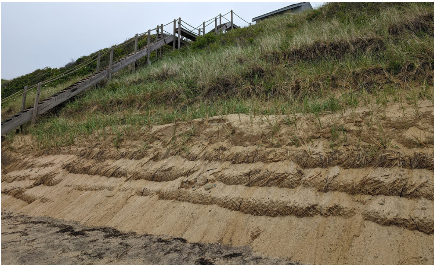
CONDITION OF EXISTING FIBER ROLL ARRAY; MANY ROLLS ARE DETERIORATING OR SHIFTING.
