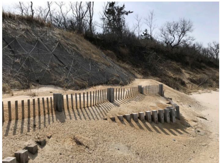
AFTER MAJOR STORMS, THE FENCE MAY NEED TO BE COVERED WITH NOURISHMENT
